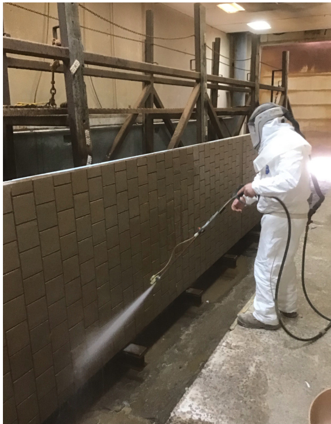
Photo 6: Applying Acid to Brick Embedded in a Precast Concrete Panel
